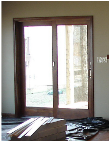
Sliding doors (3 sliding doors)
