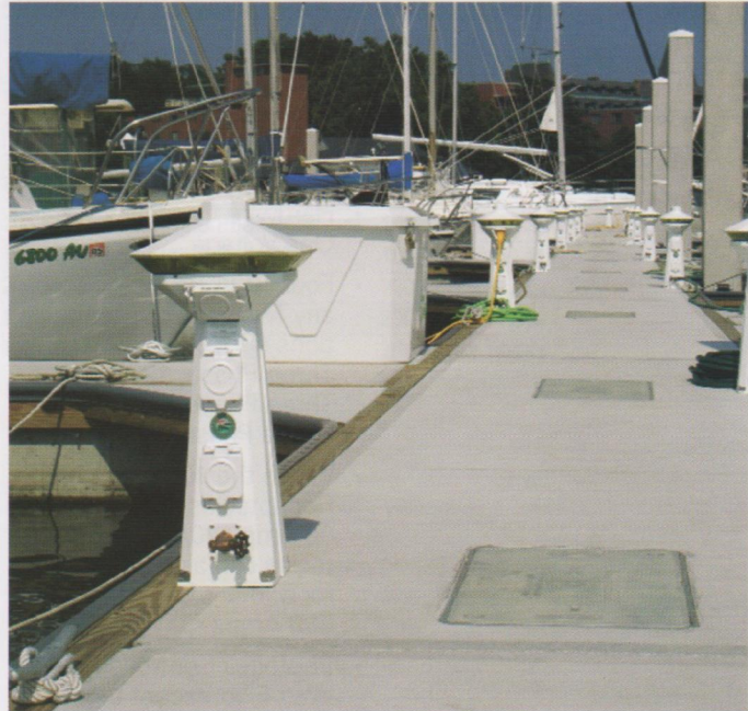
Above: Hatteras Light Power Pedestals
